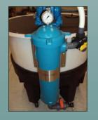
BAG FILTRATION FOR SEPARATING SOLIDS FROM DISCHARGE WATER.
